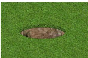
A hole is prepared in the required place in the ground (the hole should be about 80mm larger than the diameter of the box itself, eg for type STAKOHOME-7702-A it is a hole approx. 250mm, as this type has a box diameter of Ø 170mm) and the appropriate cables are fed.
